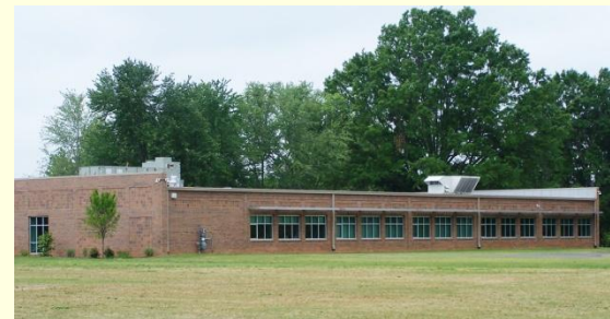
New classroom additions at Wren Middle.
